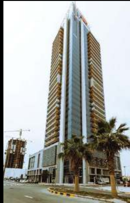
Al Manarah Tower JVT Dubai
