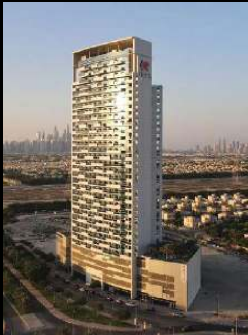
Al Jawahara Tower JVT, Dubai
